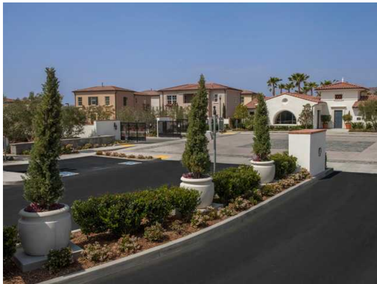
Community Center at the Villa Metro community on Soledad Canyon Road in Santa Clarita, across from the Metrolink station. Robert Hidey Architects/courtesy photo
